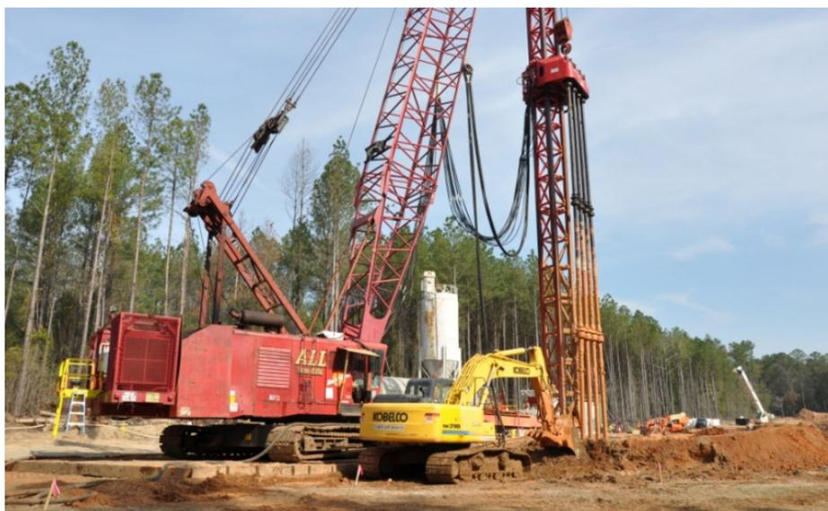
Installation of funnel and gate controls for groundwater treatment
